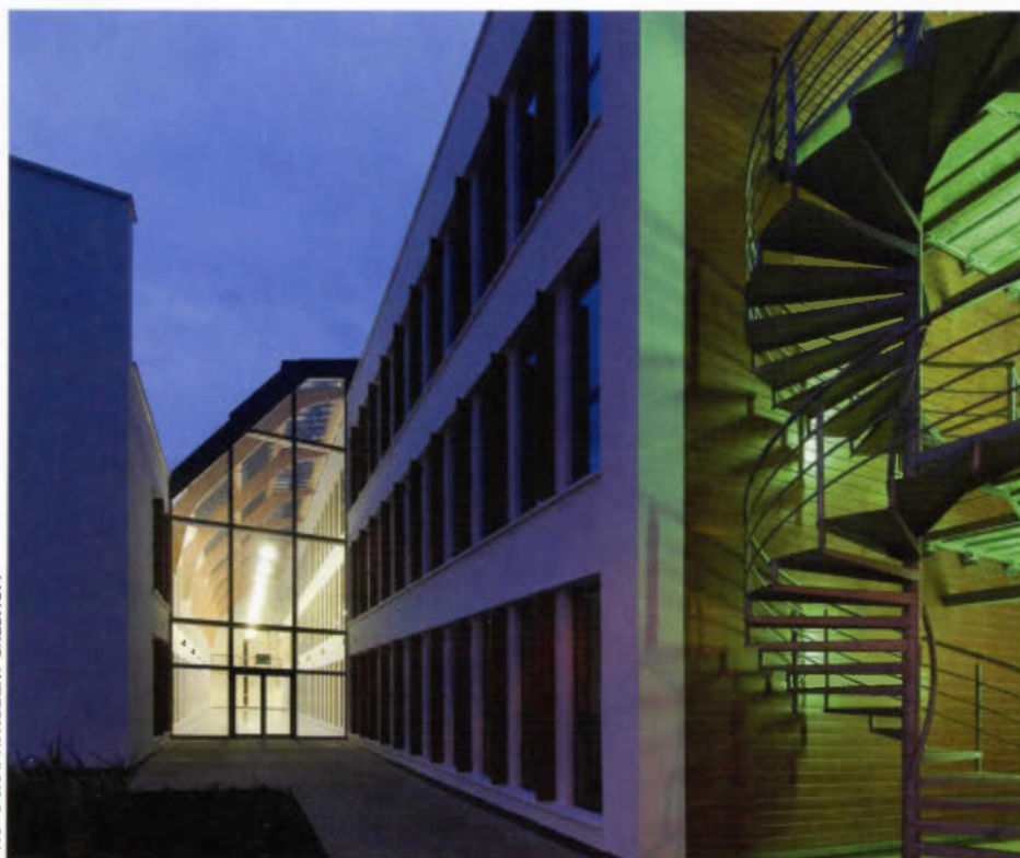
Left: The glazed "street" between the two blocks helps to achieve a 4.5% average daylight factor in the offices.
