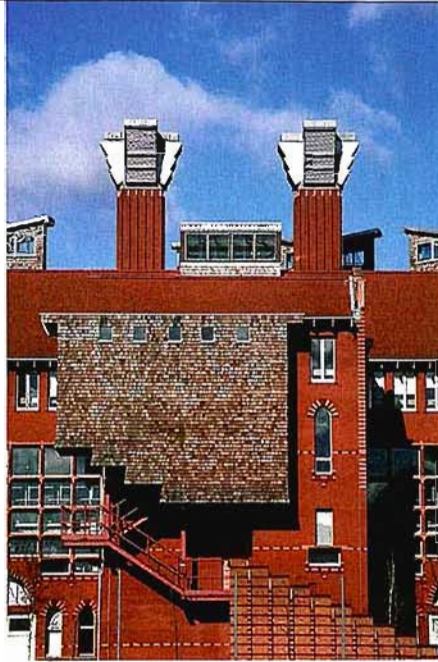
The Queens Building at De Montfort University was designed by Short Ford Architects with Max Fordham LLP as environmental engineer. It is designed to be naturally ventilated and daylight, the results being explicit in the architecture. The tall chimneys provide natural ventilation for the lecture theatres..
